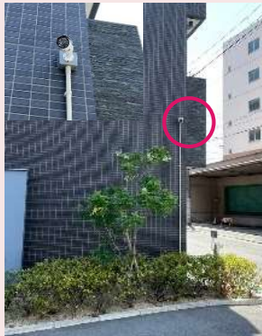
Security camera installation (Artiza Awajieki-higashi, etc.)
