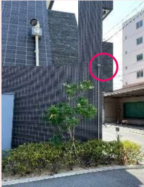
Security camera installation (Artiza Awajeki-higashi, etc.)
